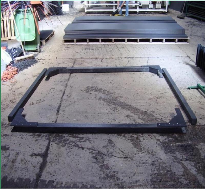
1. Lay floor/ base flat on the ground. Depending on the size of your ark, there may be some assembly required to complete. You will need to screw it all together. There are countersunk holes in the brackets to show where screws are required.
