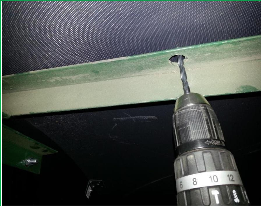
23. Again, from the inside of the ark drill up through the top, central metal bar through the top of the roof. There will only be 2 holes on the bar. It is easier to use a smaller drill first followed by a larger 16mm drill bit.
