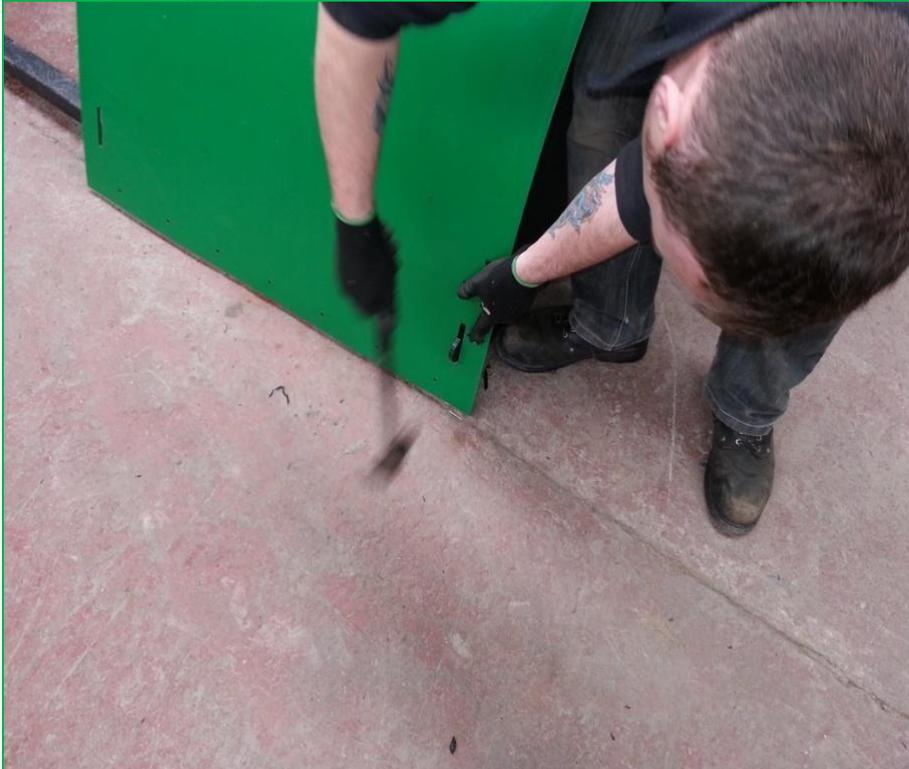
13. Once the roof is in place and it is just the final, small lug left to slot through, a hammer will probably be needed to knock the roof flat against the front/ back.
