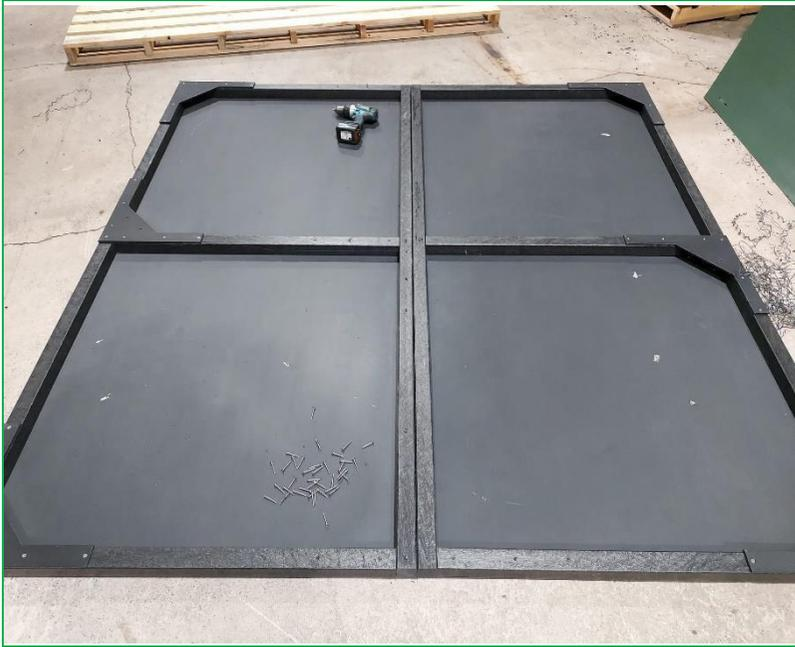
1. For a Solid Floor, lay the Stokbord floors flat on the ground with the profile side up and place next to each other.
