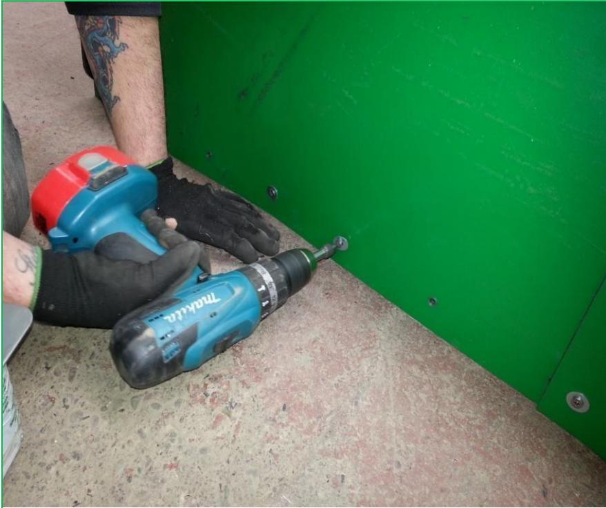
19. Using the pre-drilled holes along the base of the roof drill the screws in place using a washer.
