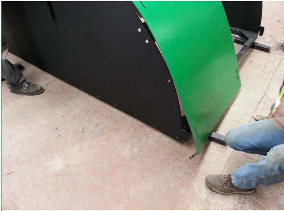
11. Lay the roof over the top of the ark ensuring that your chosen colour is facing upwards. The outside edge will have slots for the lugs on both the front and back to come through. (8ft x 4ft roofs will have slots on both sides of the panel) Putting blocks, a brick or a piece of wood underneath the floor at this point will make slotting the roof in easier.
