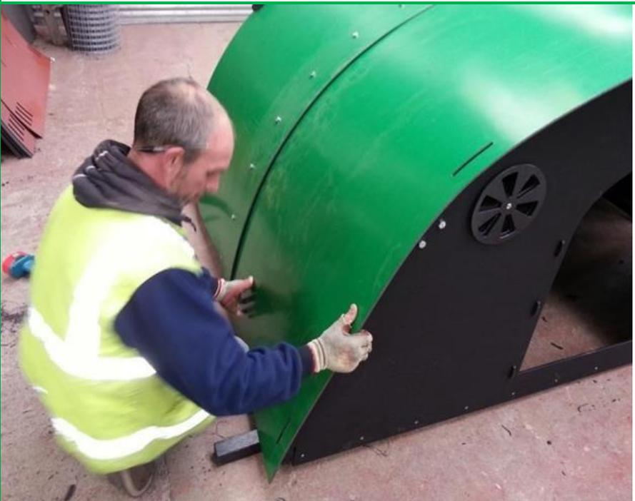
16. Place the second roof panel over the pig ark repeating the process followed with the first panel.
