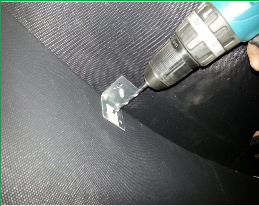
21. For the next part you have to physically climb inside the pig ark. The metal angles previously attached to the inside of the front and back are to be connected to the roof panels.
