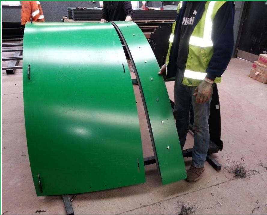
15. Slide the central joining strip into position. The roof panel that is in place will slide into the centre of the joining strip. Make sure this is tight over the roof panel and flush with the panel ends.
