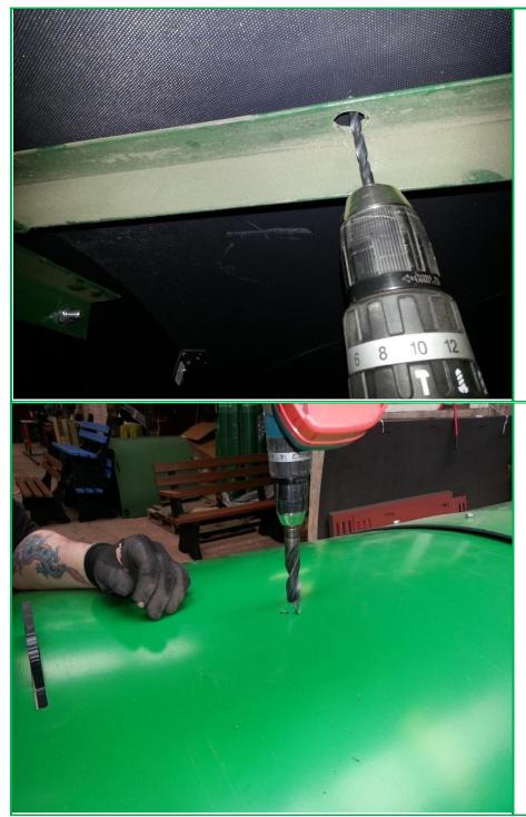
23. Again, from the inside of the ark drill up through the top, central metal bar through the top of the roof. There will only be 2 holes on the bar. It is easier to use a smaller drill first followed by a larger 16mm drill bit.
