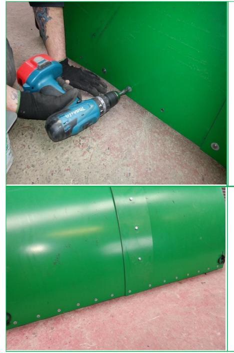
19. Using the pre-drilled holes along the base of the roof drill the screws in place using a washer.
