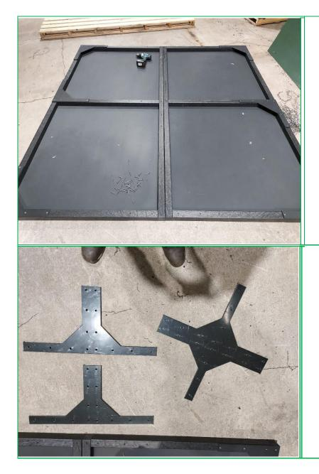
1. For a Solid Floor, lay the Stokbord floors flat on the ground with the profile side up and place next to each other.
