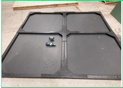
1a. There are 3 brackets to screw both floors together. Now flip the floors over and you are ready to build.
