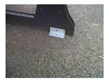
Screw the Solway brackets into the legs with stainless steel screws. Make sure all the legs are still square and then mark and drill the hole into the ground before fixing.
